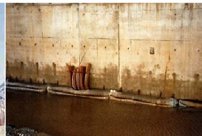
Figure 18 – Grout Bag Foundations
