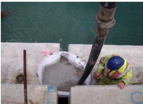
Figure 28—Shear Key
