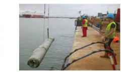
The lower construction thickness of concrete mattress provided a cost effective solution and importantly minimised the span height of the quay wall and maximised its protected embedment depth.
