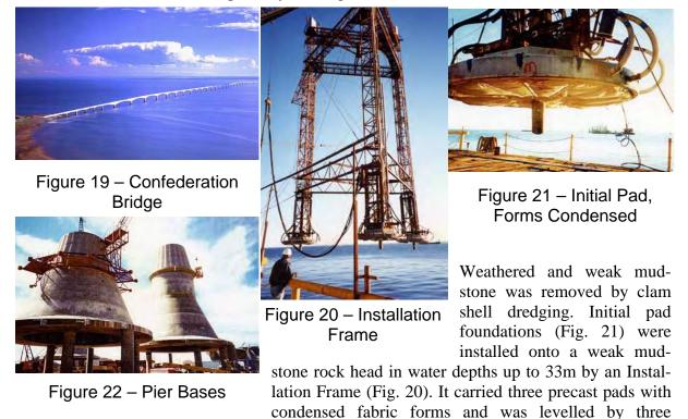
hydraulic rams. The Installation frame was fully automated for levelling, grout filling, vent monitoring and removal. Divers were only required to undertake monitoring duties. The hard pads were each formed in 5 compartments to limit risks of local failures, and were filled with a neat cement grout including an anti-shrink additive. Fig 30 shows an initial hard pad trial.
