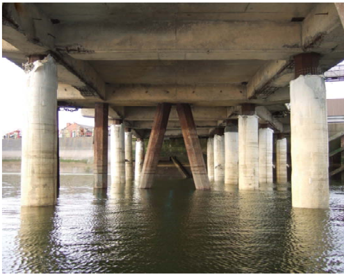
Fig. 27 – Jetty Pile Repairs
