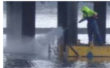
Fig. 9 – Jet Cleaning
