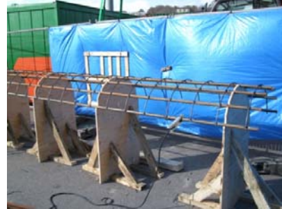
Fig. 6 – Reinforcement Cage
