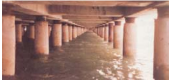
Fig. 16 – Encased Piles
